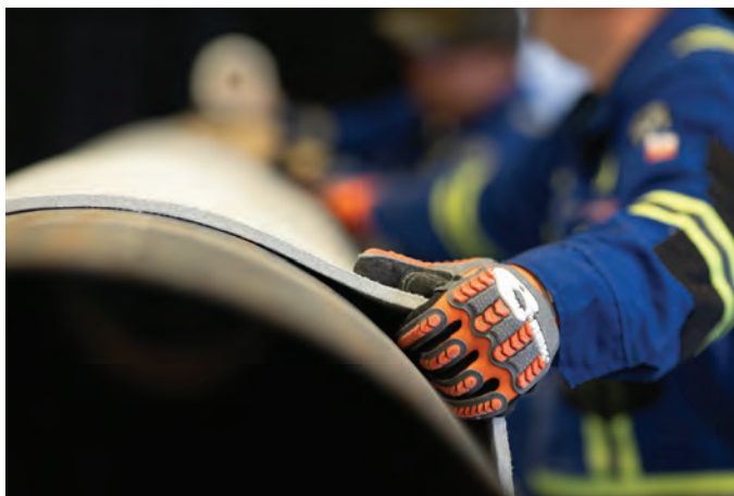
Figure 5. AlkeGel is a flexible insulation blanket providing low dust and ease of installation.
