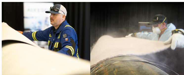
Figure 6. AlkeGel installation: minimal dust (left), and traditional aerogel blankets: extreme dust (right).
