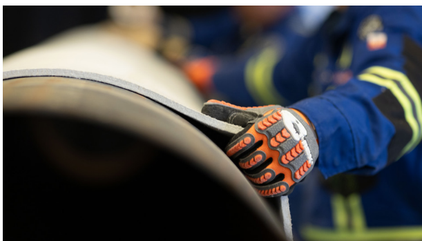
Figure 3. AlkeGel insulation blankets are lightweight, easy to handle, and install 20% faster than traditional aerogel blankets.
