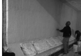
Application on ceramic fiber modules
